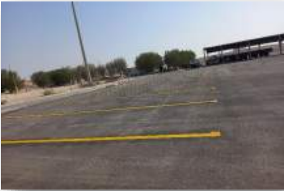
DFTC ASPHALTING WORK at DHAHRAN SAUDI ARAMCO
