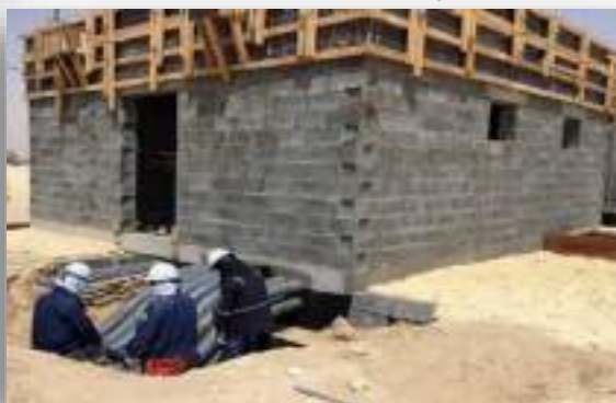
RTU BUILDING at SAFWA SAUDI ARAMCO
