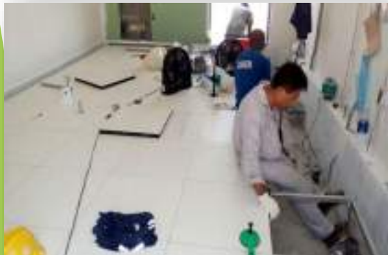
RTU BUILDING CONSTRUCT at SAFWA SAUDI ARAMCO
