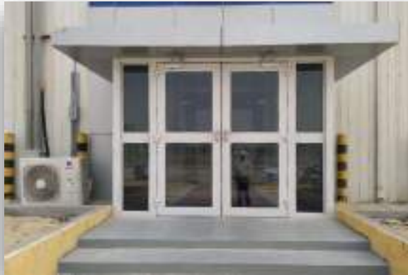
RENOVATION BLDG 9169 at DHAHRAN SAUDI ARAMCO
