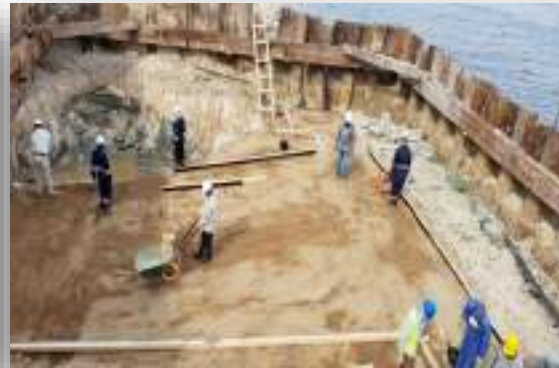
OUTFALL STRUCTURE at DURRAH , YANBU
