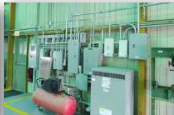
DFTC SSU RENOVATION at DHAHRAN SAUDI ARAMCO
