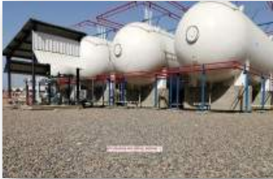
OVERHEAD TANK INSTALL at DURRAH , YANBU
