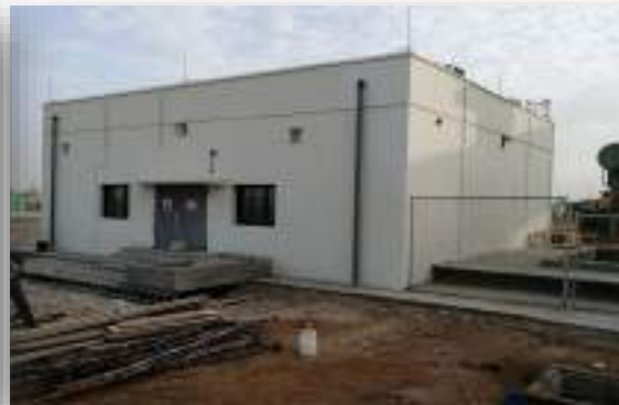
BUILDING CONSTRUCTION at DURRA, YANBU
