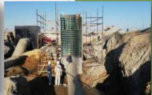
CONSTRUCTION at DURRA, YANBU
