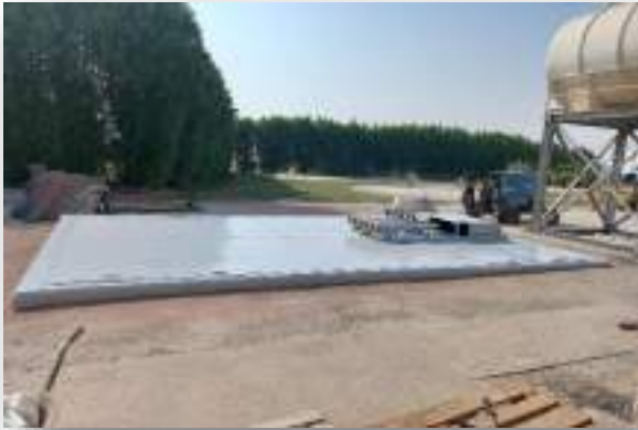
WATER TANK REPAIR at DHAHRAN SAUDI ARAMCO
